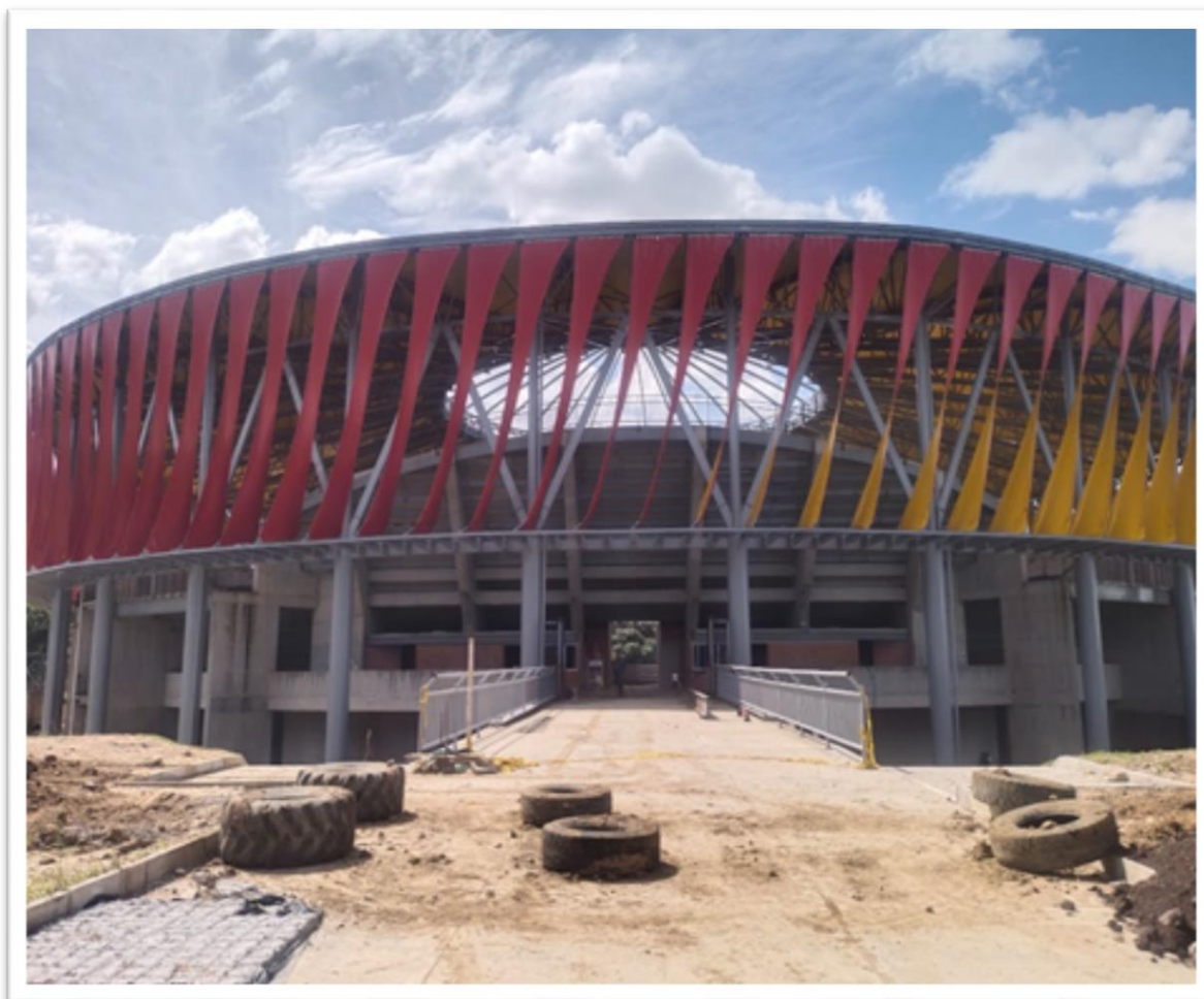
Obras coliseo mayor
